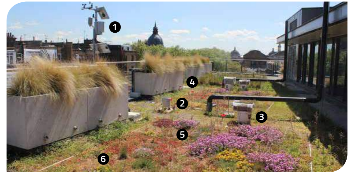
The roof is equipped with instruments to measure 1 weather conditions 2 rainfall 3 water quality 4 runoff 5 soil moisture 6 soil and roof temperature
