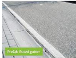
Prefab fluted gutter
